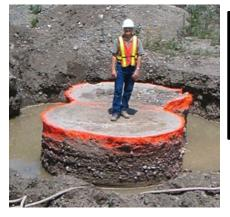
In situ soil stabilization and solidification by mixing in Cementous slury into the soil to prevent leaching over a long time span
