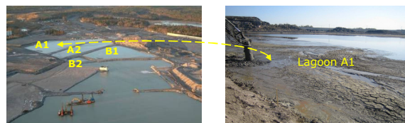
The largest mass stabilization project in Finland
