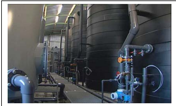
Figure 1: Bioreactor system Hoogeveen
