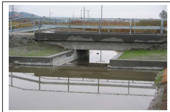
Part of culvert with wier (2005)
