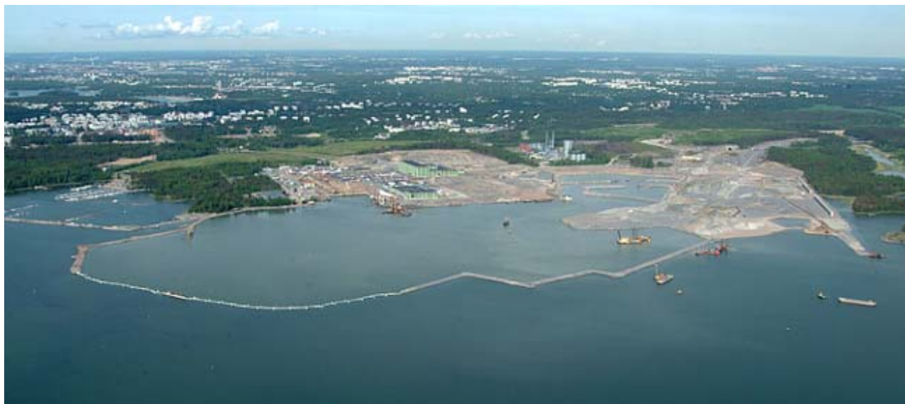
Figure 4. Decontamination dredging in progress (June 2005).
