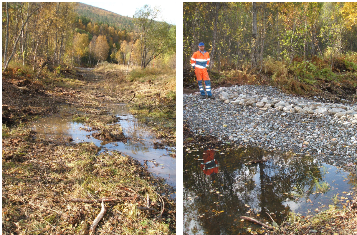
Figure 1. Wetland and threshold under construction. The threshold has an impermeable core.
