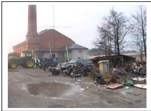
Plant site before remediation
