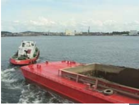
Capping, pilot project Kristiansand
