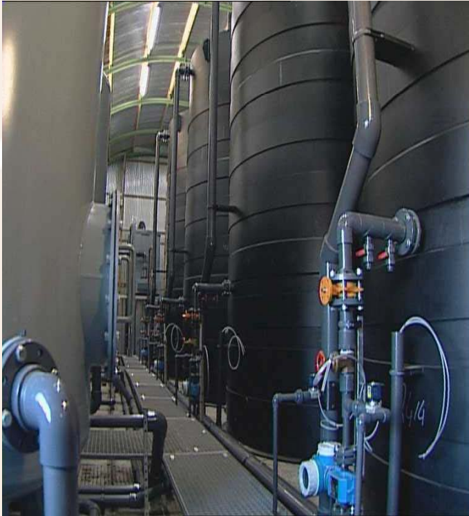
Fixed system, 100 m 3 volume
