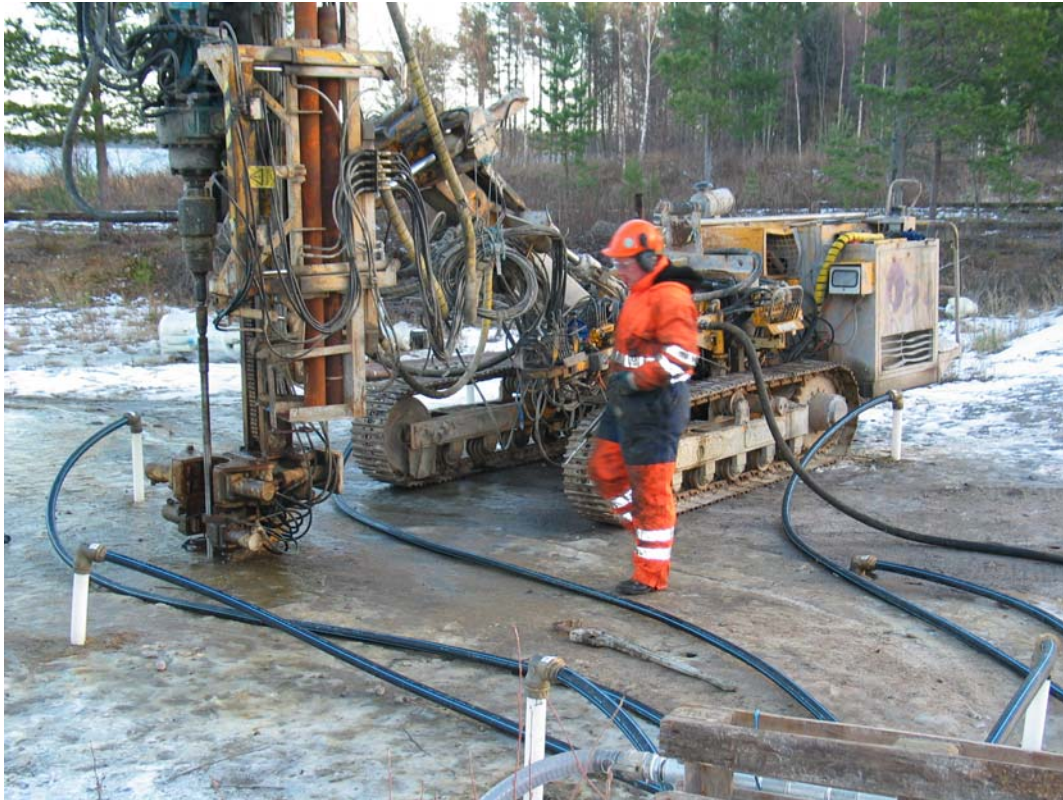
Figure 1: Injection equipment during injection
