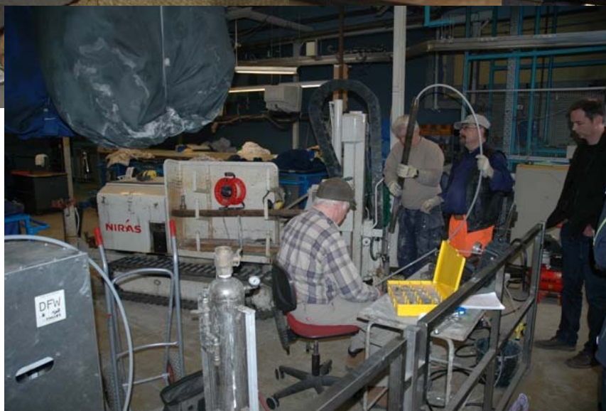
Installation af FLUTe liner
