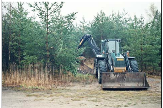
Soil sampling by digging
