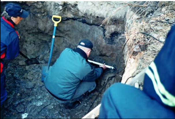
Installation of soil on-line monitoring sensors
